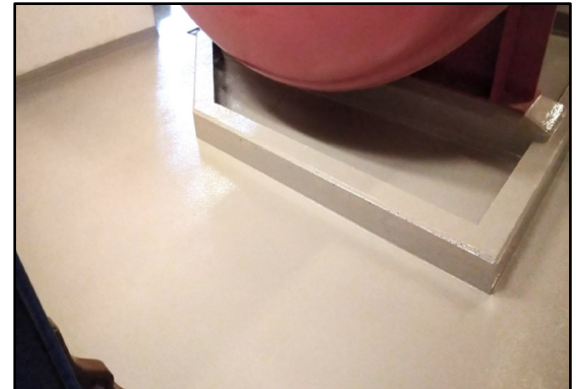
After: floor coated with ARC NVE VC.
