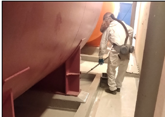
In progress: ARC NVE VC being applied.
