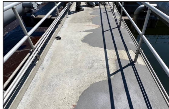
Loose and damaged concrete repaired with ARC EG-1.
