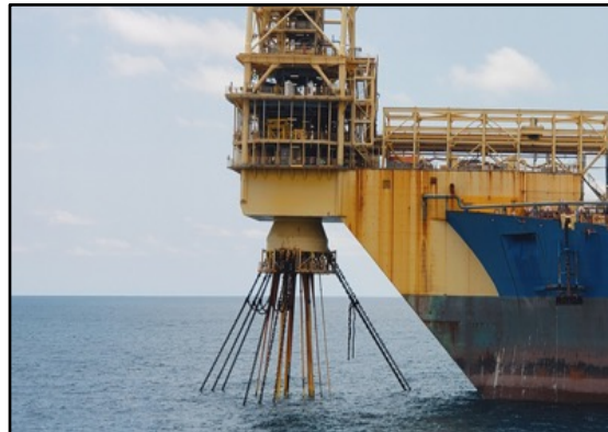
Floating Liquefied Natural Gas (FLNG) Platform.
