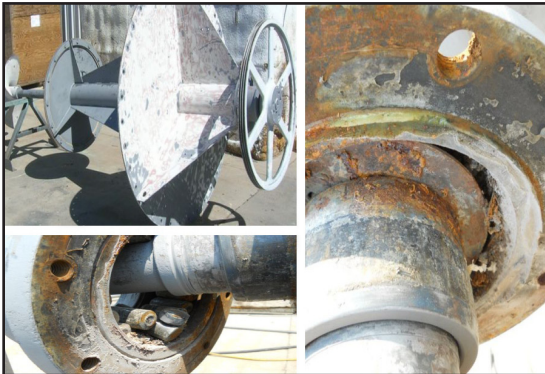
Greasing hard to seal shaft bearings was unreliable. Annual failure was expensive.
