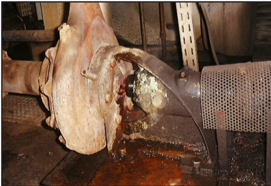
Condensate pump with Chesterton 180H Cartridge Seal.
