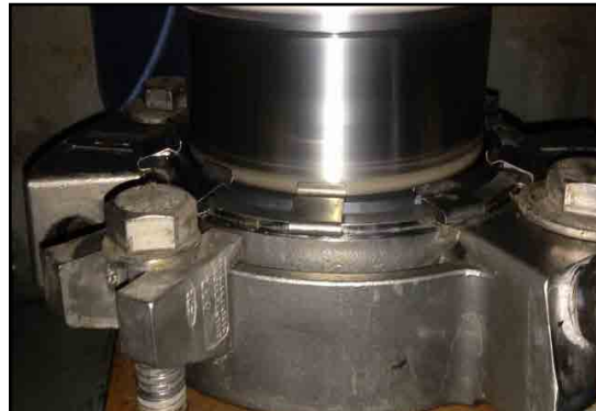
Chesterton 442 Split Seal during pump operation.
