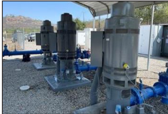
Chesterton Connect Sensor attached to pump.
