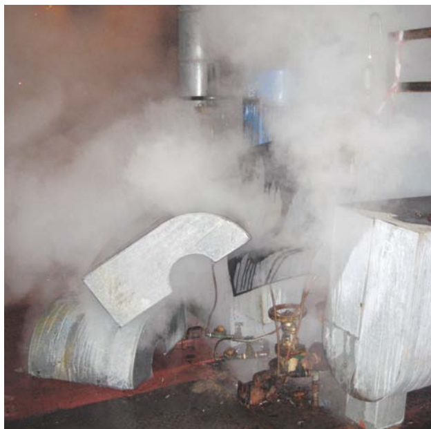
Time to fix the leak
