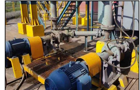
Pumps where packing was installed.
