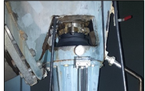
Running for almost one year without gland adjustments.
