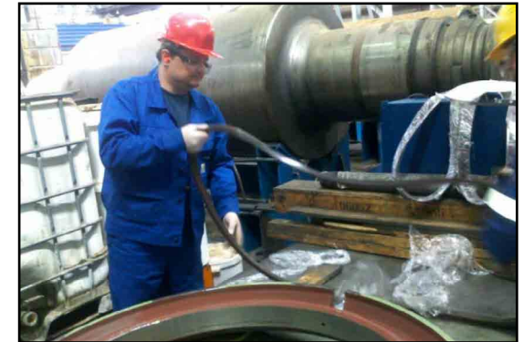
Installation of 50KWS seal
