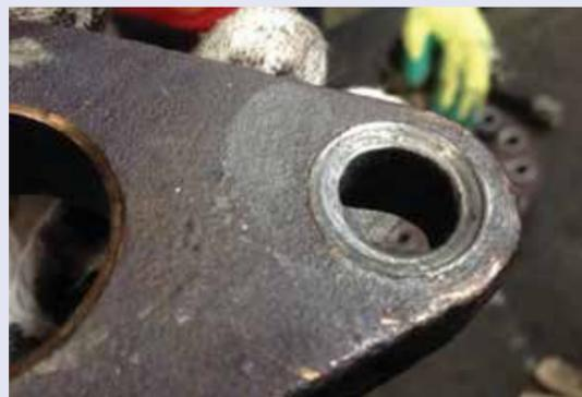
Figure 3. Inadequate Gland Flange Surface Finish and Hardness for Low Emission Sealing.
